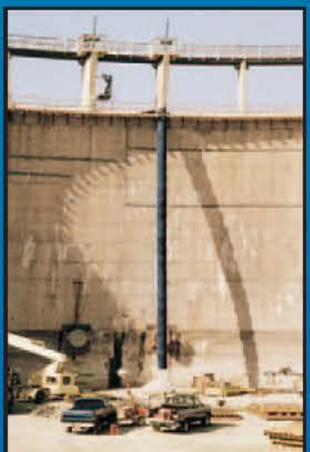
Canyon Lakes Dam, CA
